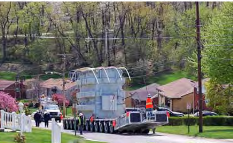
866,300 LB. GENERATOR 844,000 LB. TRANSFORMER
