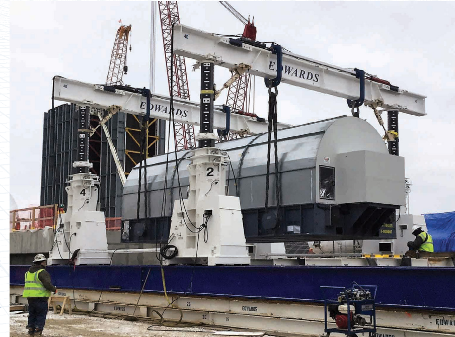
500T Gantry System moving a 756,184 lb. Gas Turbine Generator into place on site.
