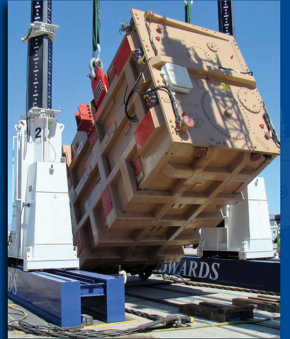
▲ 485,016 lb. transformer offloaded from rail car and up-ended at nuclear facility.
